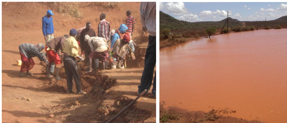
Photos: De-silting of Hula-Hula Dam (left) and dam recharged after first heavy rain falls (right)
